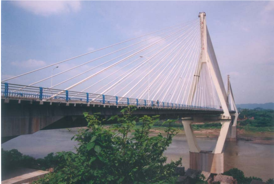
NOCX pipe white incl ext spiral on Masangxi Bridge, China
