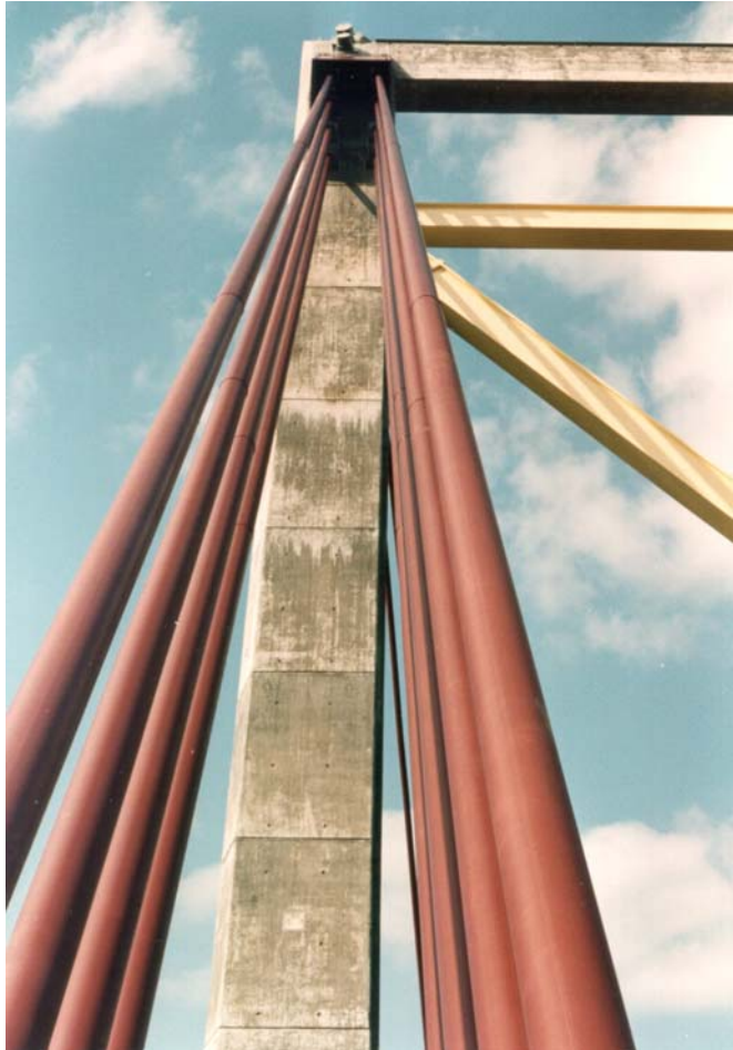
NOFX pipe red-brown on Schaffhausen Bridge, Switzerland
