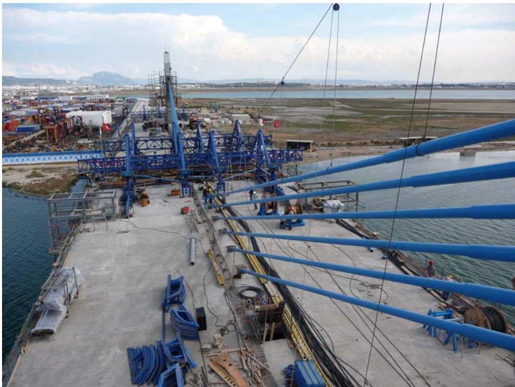
NOCX pipe blue incl ext helix on Rades La Goulette Bridge, Tunisia
