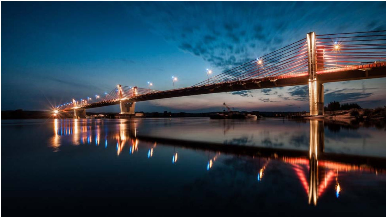
NOCX pipe red on Vistula Bridge, Kwidzyn Poland
