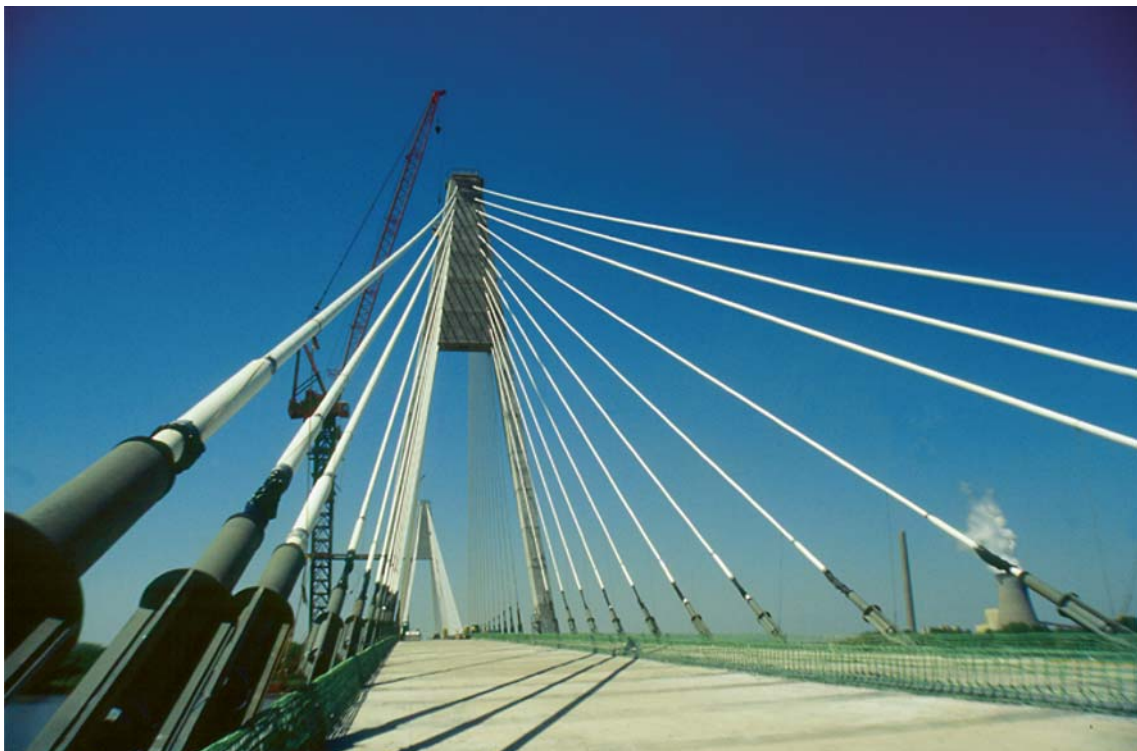
NOCX pipe white incl ext spiral on William Natcher Bridge, USA
