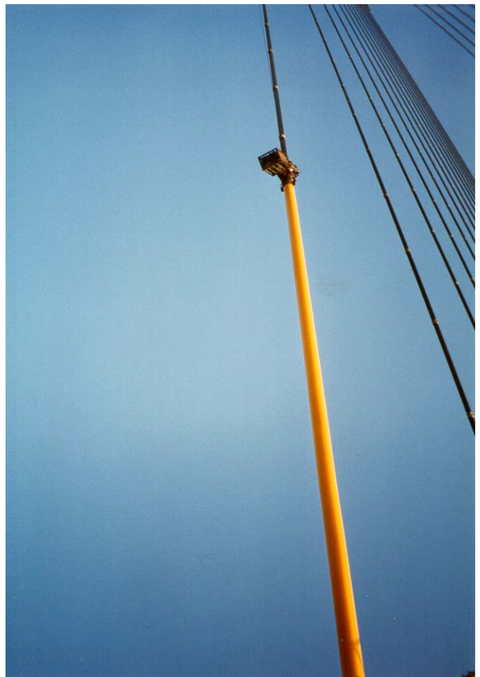
Lifting of welded half-pipes
