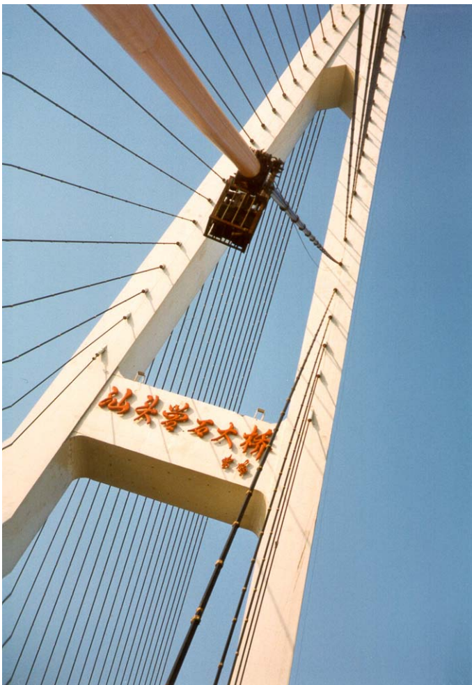
Lifting of welded half-pipes
