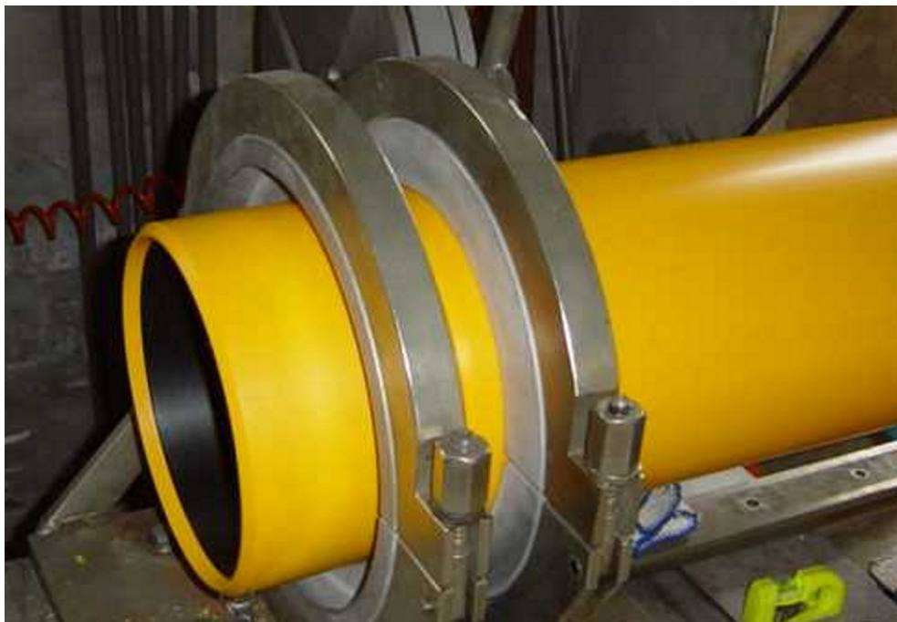
Butt Welding of Electrofusion Coupler to Pipe Sleeve
