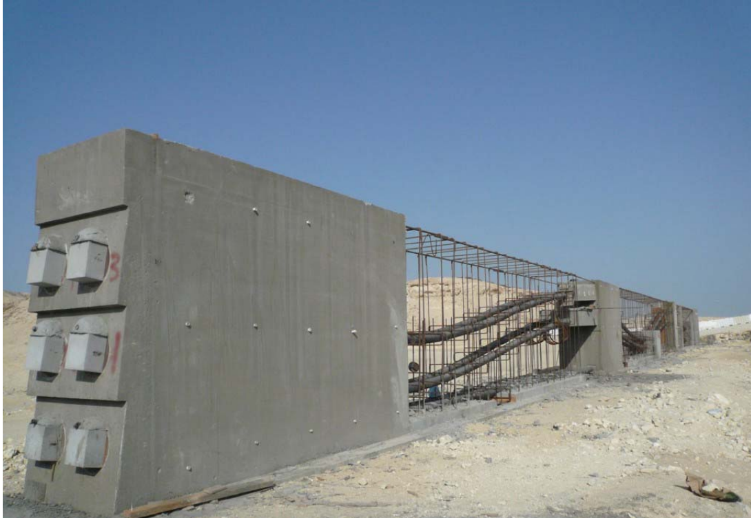
IP 4 M PE Duct Full 37 m Scale Trial
