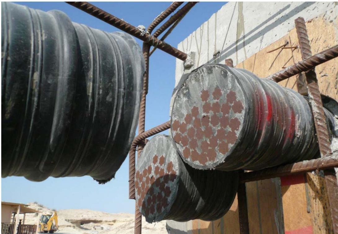
IP 4 M PE Duct Detail on Full Scale Trial
